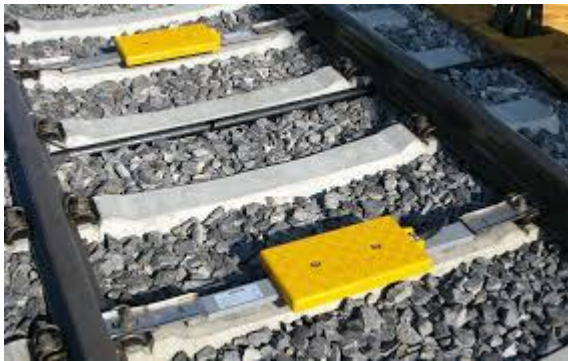
Figure 2: balises (source: Vortok Balisen Mounts ERTMS October 2008)
